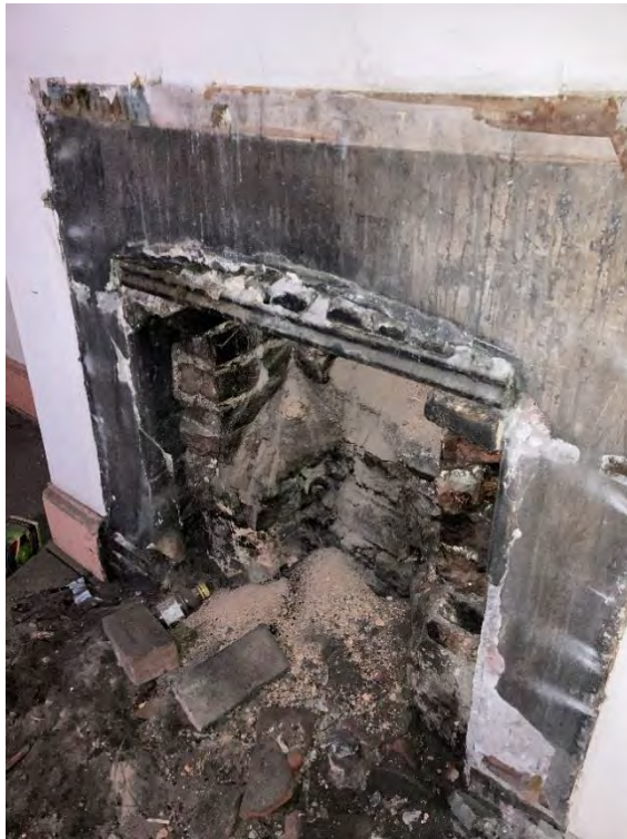
Figure 70: Fireplace in the living room with broken mantel and surround.
