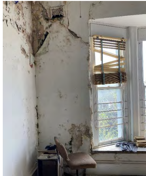
Figure 44: Dampness along the internal walls with peeled-off plaster.
